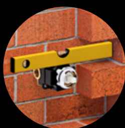
Leveling of the concealed part.
